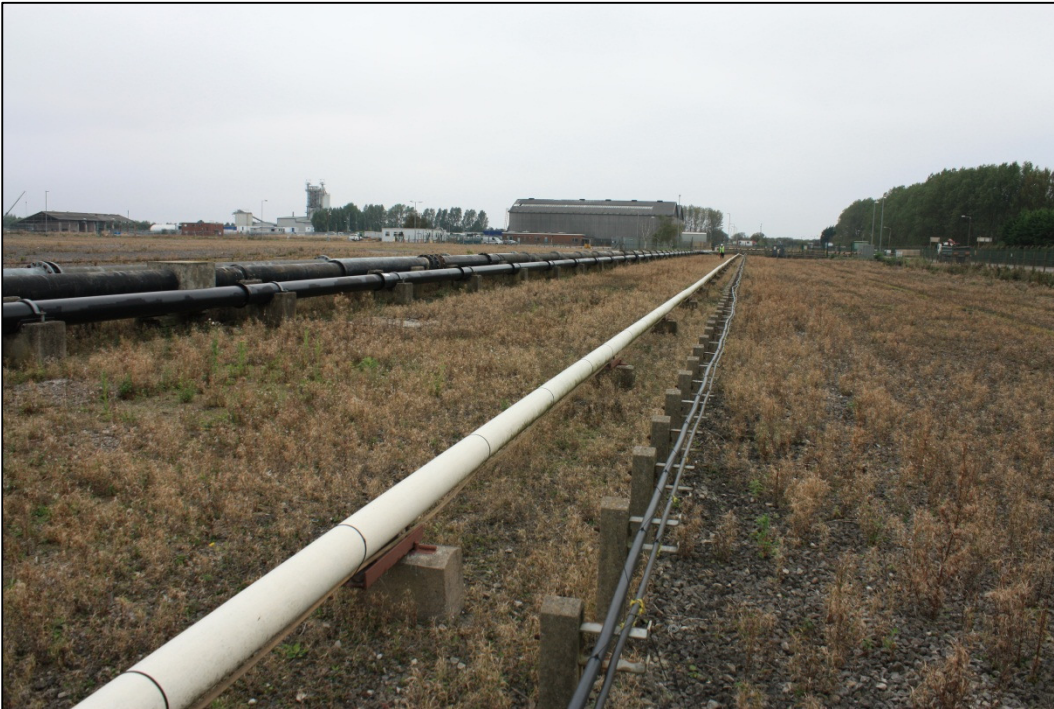
Photograph 3: Photograph located in the north of the Site, facing west along the northern boundary
